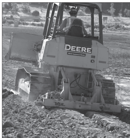
Ripping of severely compacted soils on contour for seeding purple needlegrass ( Nassella pulchra ) following construction. “Compost overs” were incorporated prior to seeding.
